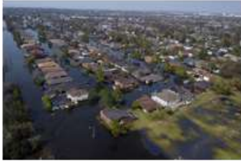
inundation (flooding): X feet (from GIS flood plane analysis)
