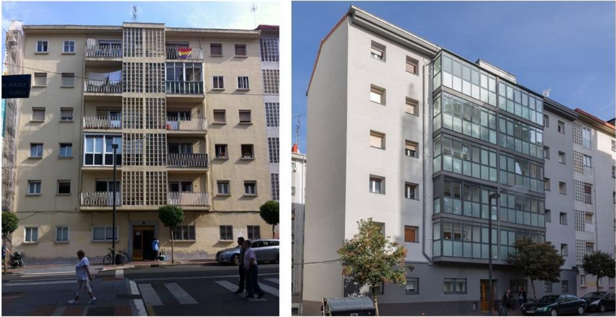
Figure 3. Apartment block before (left) and after renovation (right).
