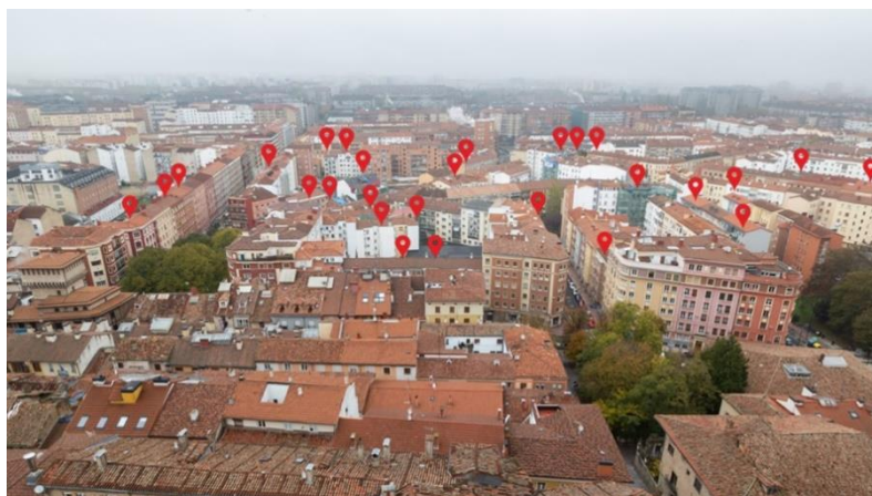
Figure 2. Detailed aerial view of the buildings that are part of the intervention.
