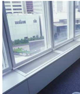
Figure 2.10b. Air Supply Swindow (View and detailed crossection)
