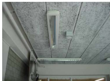
Figure 10-52. New lighting installation.
