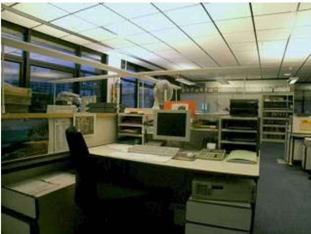
Figure 10-27. Indirect luminaire integrated in the furniture.
