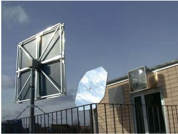
Figure 5-29. Pictures from an Arthelio project installation in Berlin. The heliostat on the roof supplies the light pipe with concentrated sunlight (left). An electrical light source supplies the light pipe with electrical light when needed (right).
