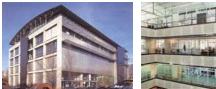
Figure 10-23. Office building, Lyon, France. Third floor offered open and individual spaces for the tests.
