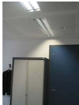
Figure 6-33 . Luminaire with daylight sensor.
