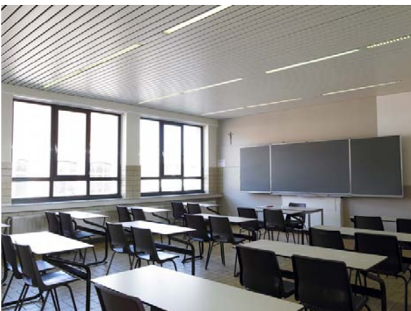
Figure 10 -74. Photo of classroom before refurbishment.
