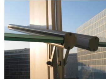
Figure6-44. Louvresinlightpenetration mode–110°slope.
