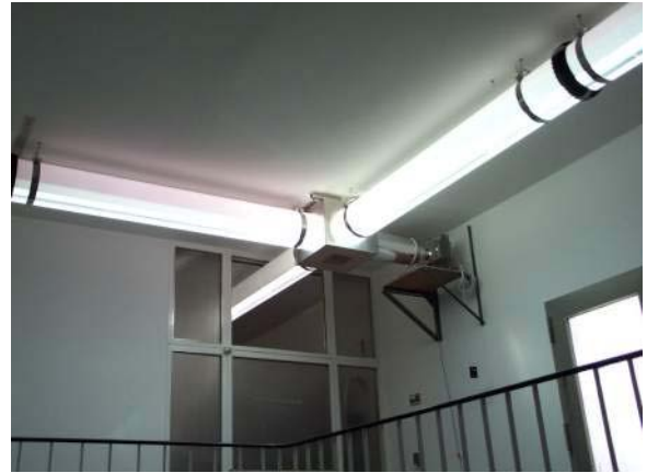
Figure 5-29. Pictures from an Arthelio project installation in Berlin. The heliostat on the roof supplies the light pipe with concentrated sunlight (left). An electrical light source supplies the light pipe with electrical light when needed (right).
