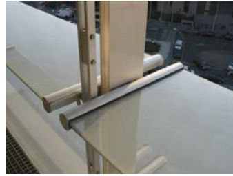
Figure6-43 . Louvresinhorizontalposition–90°slope.
