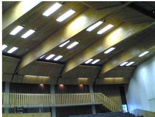
Figure 10-94. Picture before the retrofit.
