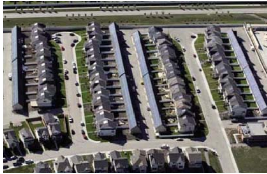
Figure 7.19: Okotoks complex (Canada).
