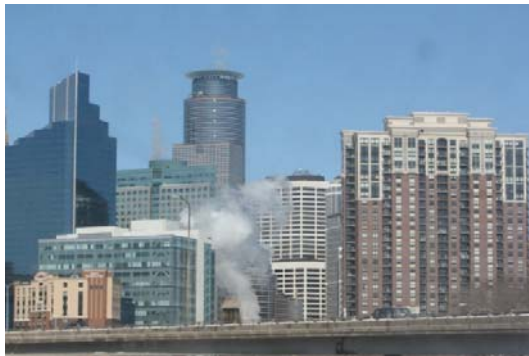
Figure 7.28: Minneapolis District Energy Cooling System Cooling Tower - Winter Operation.
