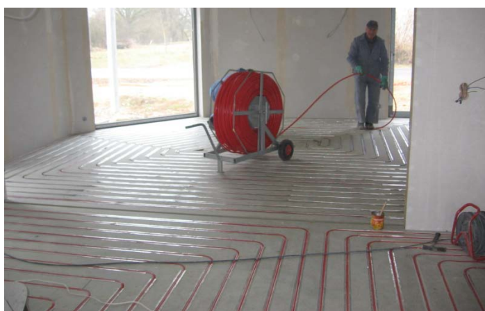
Figure 15-5 : Installation of the low inertia heating floor system
