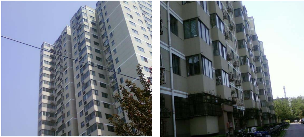
Figure 18-2. The outside view of the investigated building
