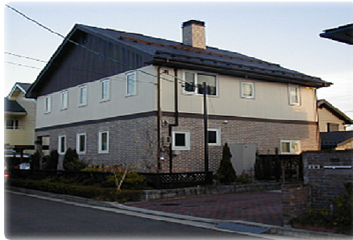
Figure 3-4. An outside view of the residence
