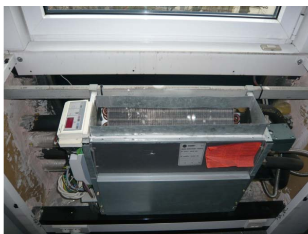
Figure 2-21: Concealed vertical fan coil unit
