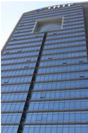
Figure 6-3: Several external windows can be opened manually of CHN-03
