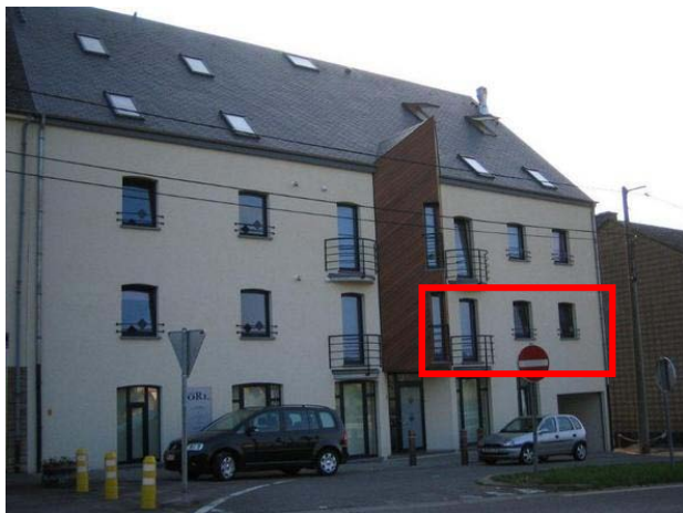
Figure 16-2 : General view of the building
