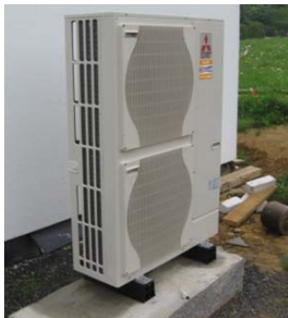
Figure 15-6 : External unit of the air-to-water heat pump
