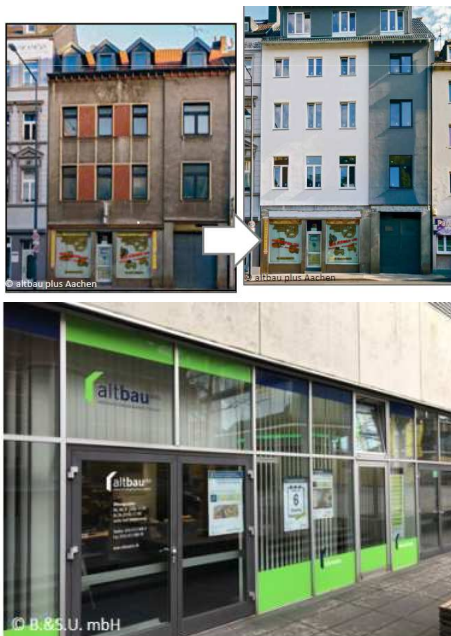
Top: Renovation of an old building by private owners in Aachen (source). Bottom: Office of the network altbau plus offering free consulting (source).
