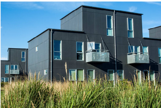
Top: Aerial photo of the district of Stenløse South (AAU, 2017). Bottom: Picture of one of the buildings in the district (AAU, 2017).
