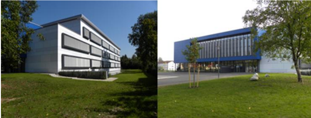
Figure 13. A picture of the renovated school building in Freilassing, Germany (Porextherm, 2012)
