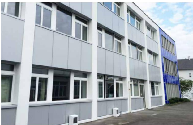
Figure 14. A picture of the renovated office building in Rheinfelden, Switzerland (Evonik Resource Efficiency GmbH, 2016)
