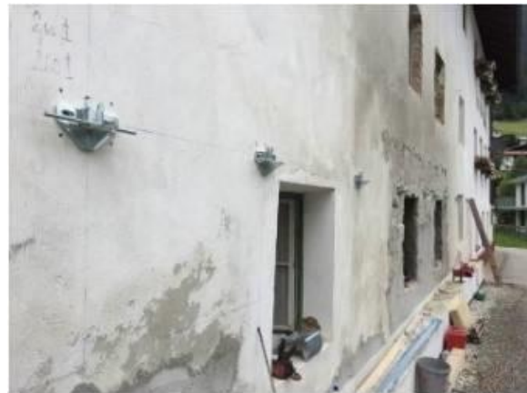
figure 157: Facade prepared with the supports for the facade, © Michael Flach
