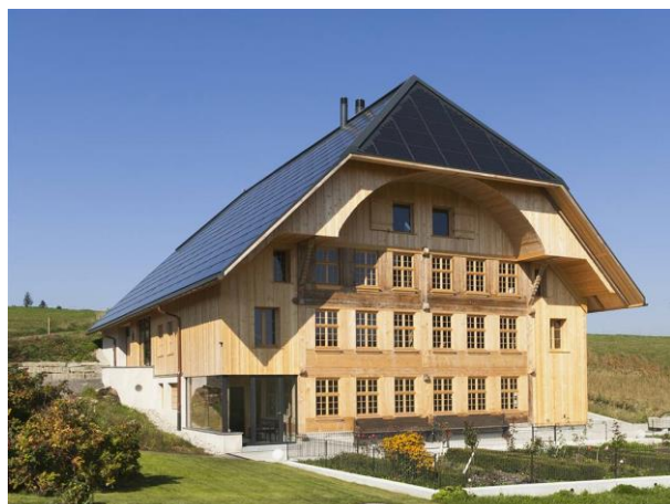
figure 176: South front after renovation © C. Anliker
