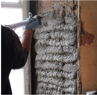
Figure 30 Spray application of insulated lime plaster © Ecological Building Systems
