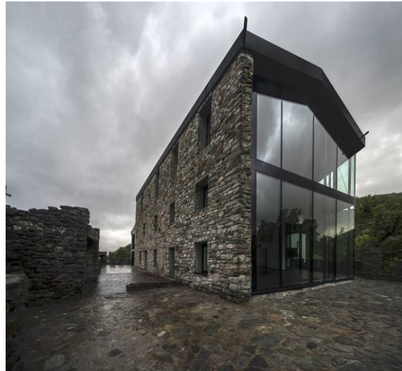
figure 57: Stone external walls © L. Carugo
