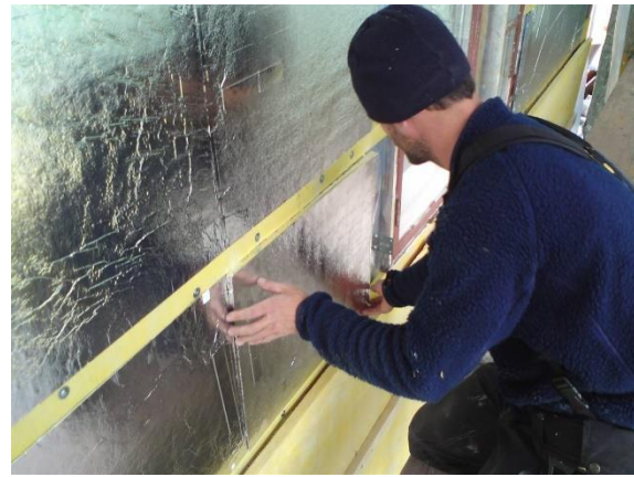
figure 113: Mounting of vacuum insulation panels, © Pär Johansson
