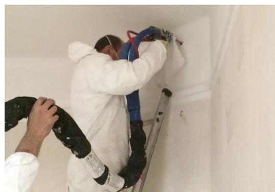
figure 87: Photograph showing the injection of the insulation foam © Gannochy Trust
