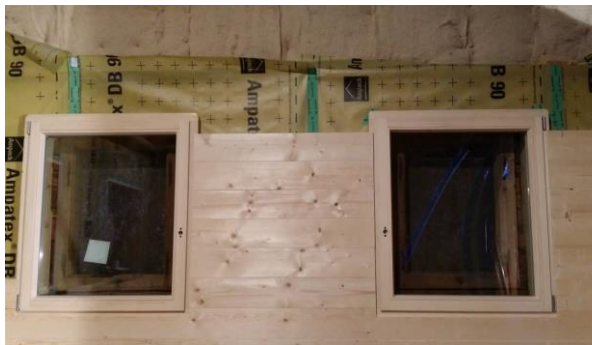
figure 72: New block wall ©Benjamin Schaller
