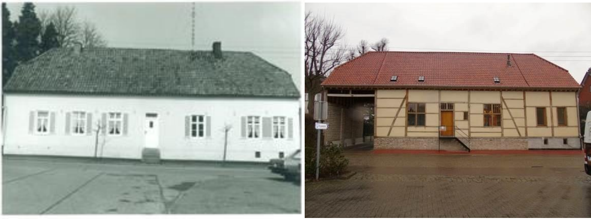
figure 181: Half timber-framed house in Alken before (left ) and after (right) restoration in 2016.
