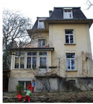
figure 79: External wall after and post intervention. © M. Hutterli
