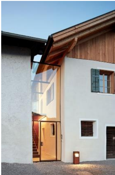
figure 29: Detail of the front of the renovated building © René Riller
