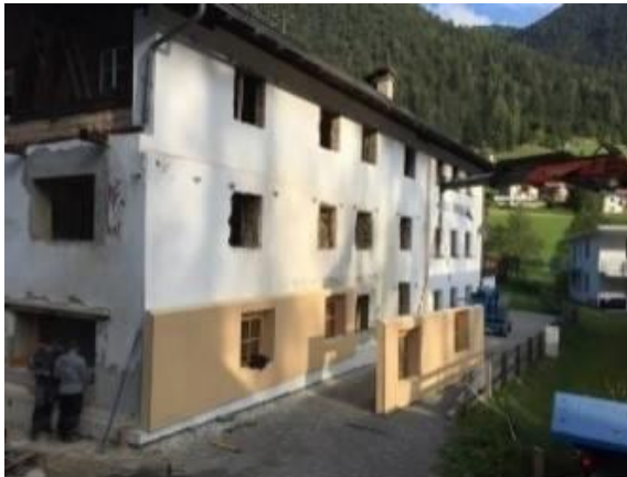
figure 156: Facade works, © Michael Flach
