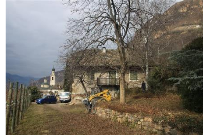
figure 25: Side of the building pre renovation © Eurac
