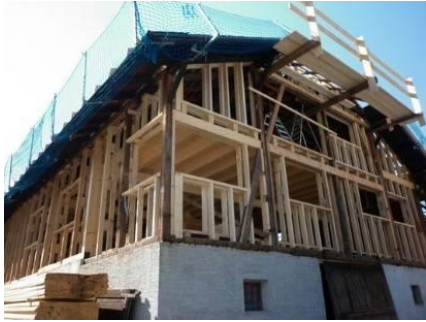
figure 167: Construction phase, © Familie Schmölz
