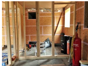
figure 67: View of the airtight surface (OSB board) © DI Hans Peter Gruber
