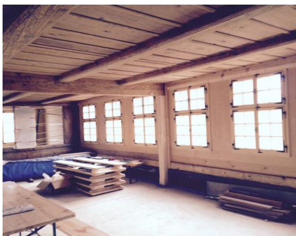
figure 173: South facade from inside during work © C. Anliker
