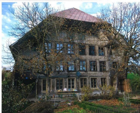
figure 175: South front before renovation © C. Anliker
