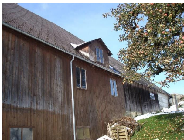
figure 174: East front before renovation © C. Anliker
