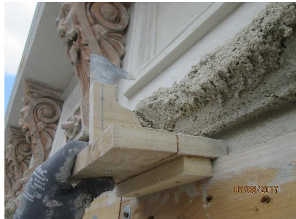
figure 129: Impressions from the work on the aerosol insulated façade, © Trimmel Wall Architekten ZTGmbH
