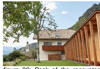
figure 28: Back of the renovated building © René Riller
