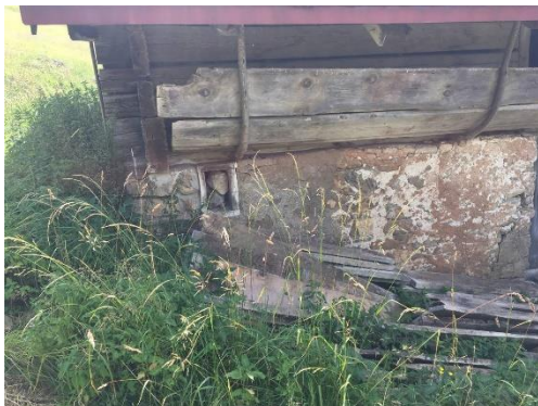
Old wall before renovation © Gehret Design
