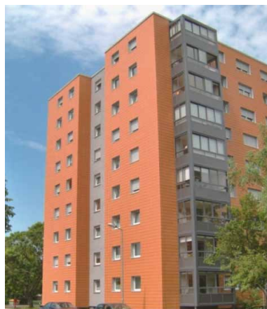
Residential building renovation in Karlsruhe, Germany.
