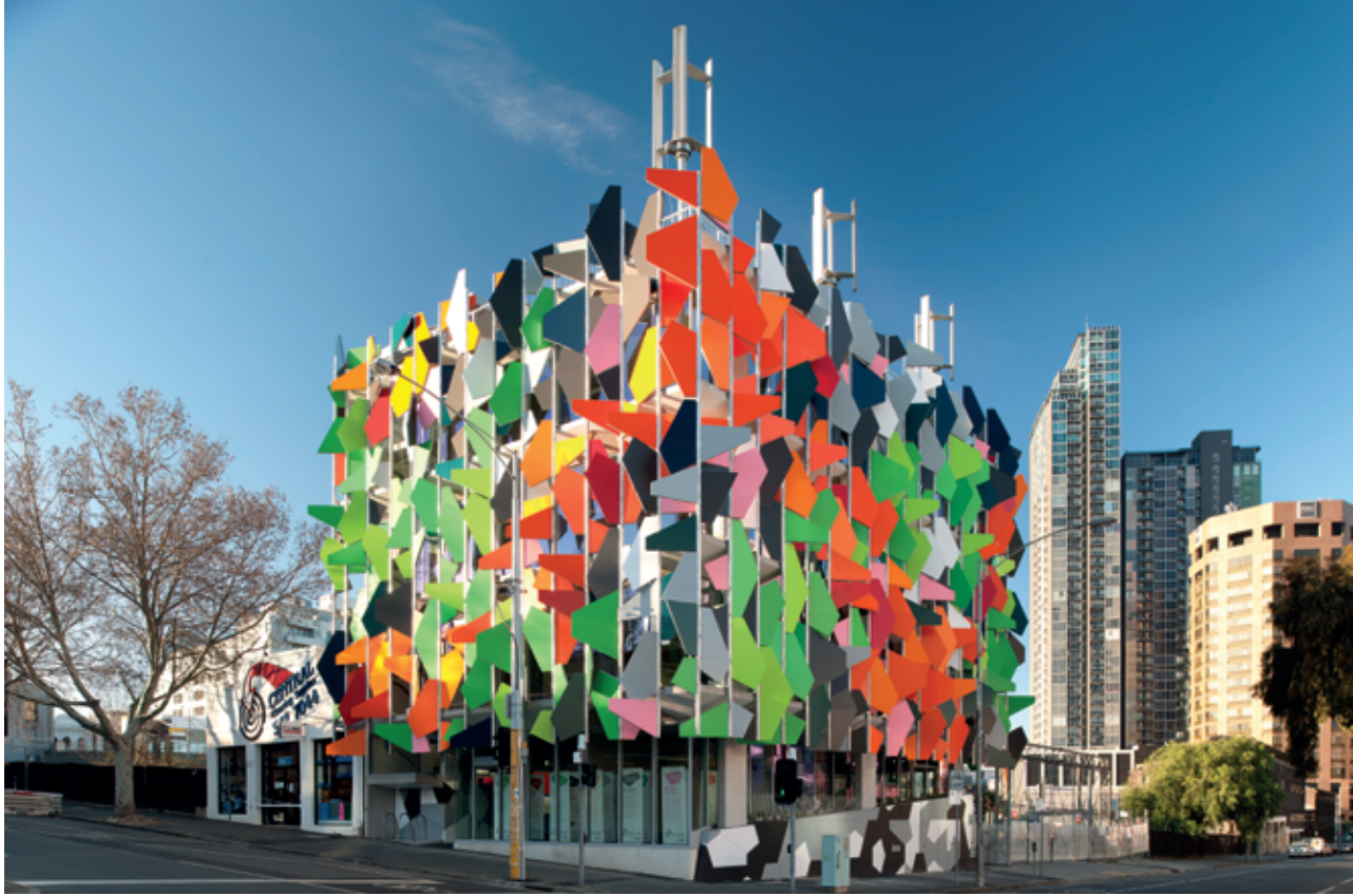
Pixel Building, Melbourne (Grocon with Studio 505 Architects). Designed for carbon neutrality, the world's highest rated Green Star and LEED building. Source: Grocon
